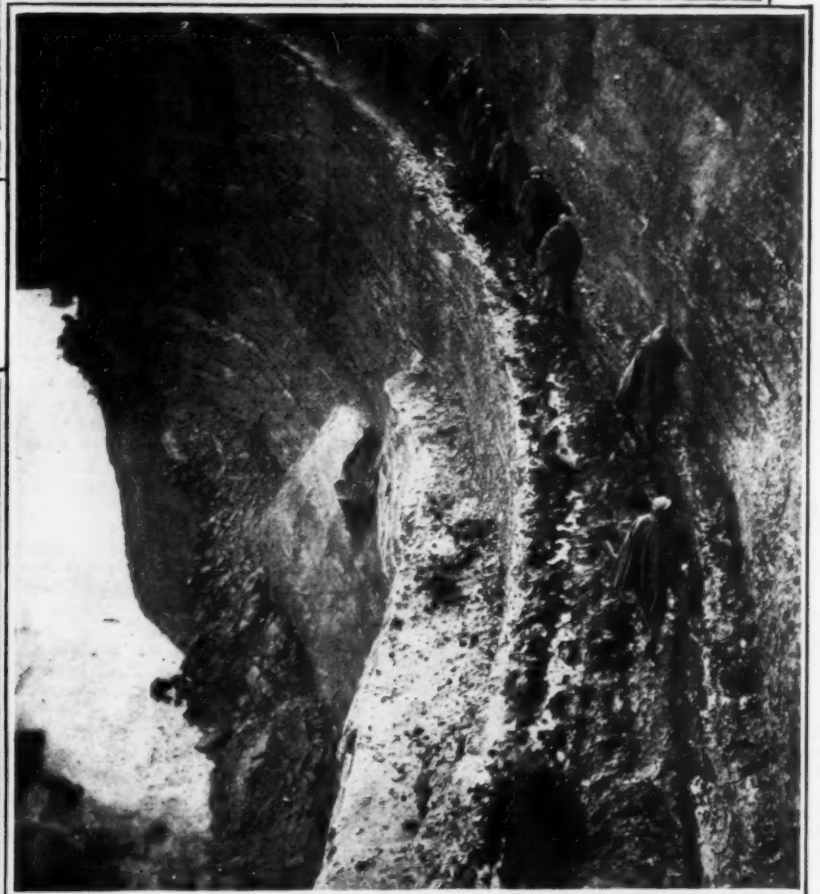
A ROAD ALONG THE EDGE OF THE ABYSS
